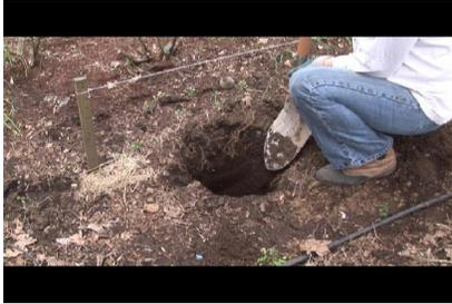
Next, you want to dig your hole for the support posts. Measure a distance of 6 feet between holes. Dig your holes 18 inches to 2 feet deep. This will ensure that your post is secure and the trellis won't tip when plants are growing up on it.
