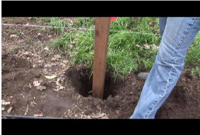
We used 10 foot treated posts that will allow an 8 foot high trellis when we are done.
