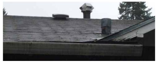
and purchase a replacement 'boot.' Place it over the vent and nail it into position using plenty of roofing tar to prevent further leaking.
